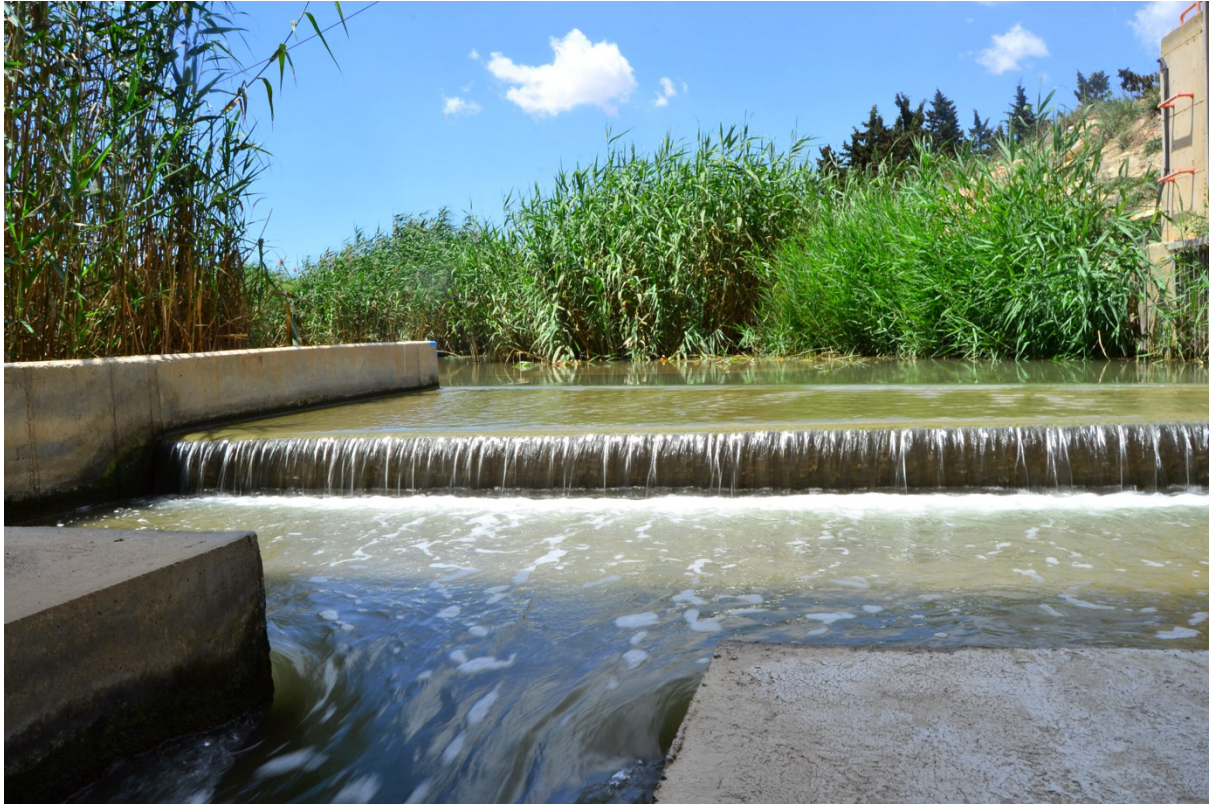
Campo de cartegena upper aquifer connected to the Menor Mar | Spain
